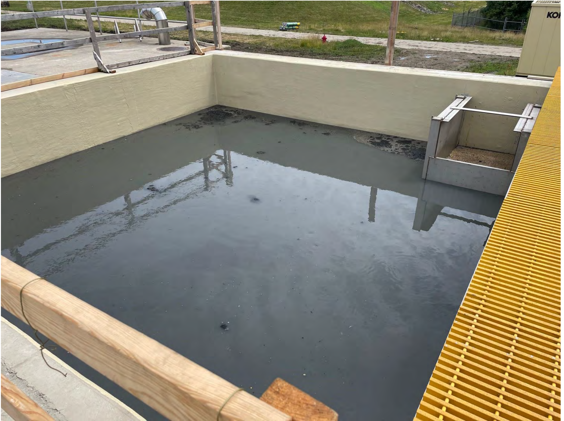
Photo 4 – East Grit Tank with new grit removal system up and running.
